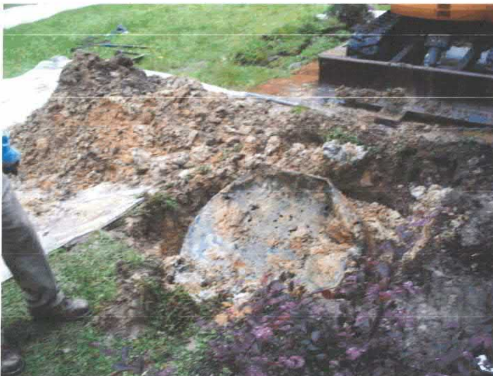
Picture 2: UST 355Ash-1 removal in progress.
